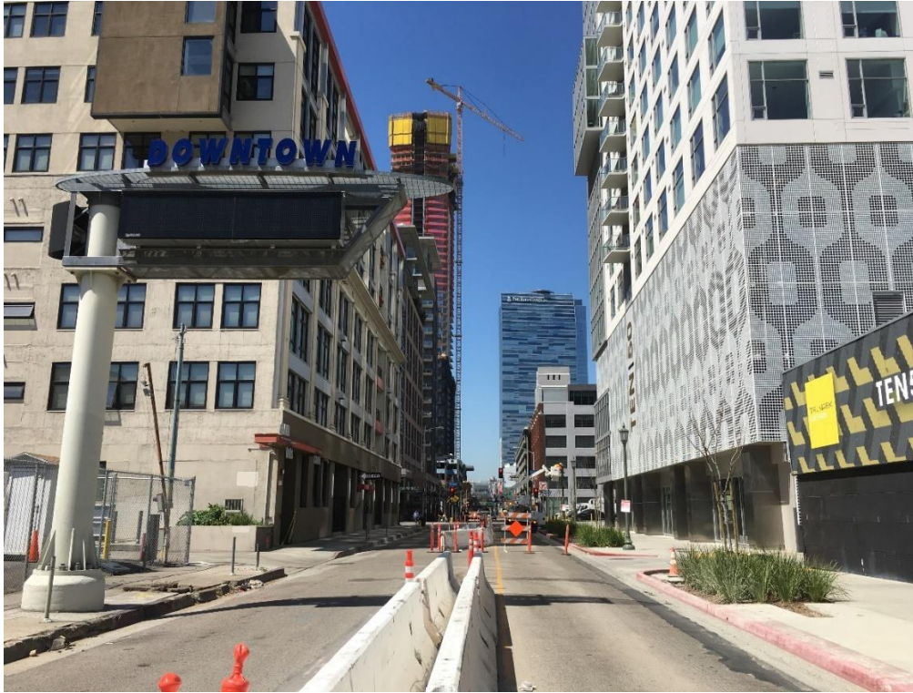
Photo 13. View of 11 th Street and adjacent signage to the project site. (Facing North West).
