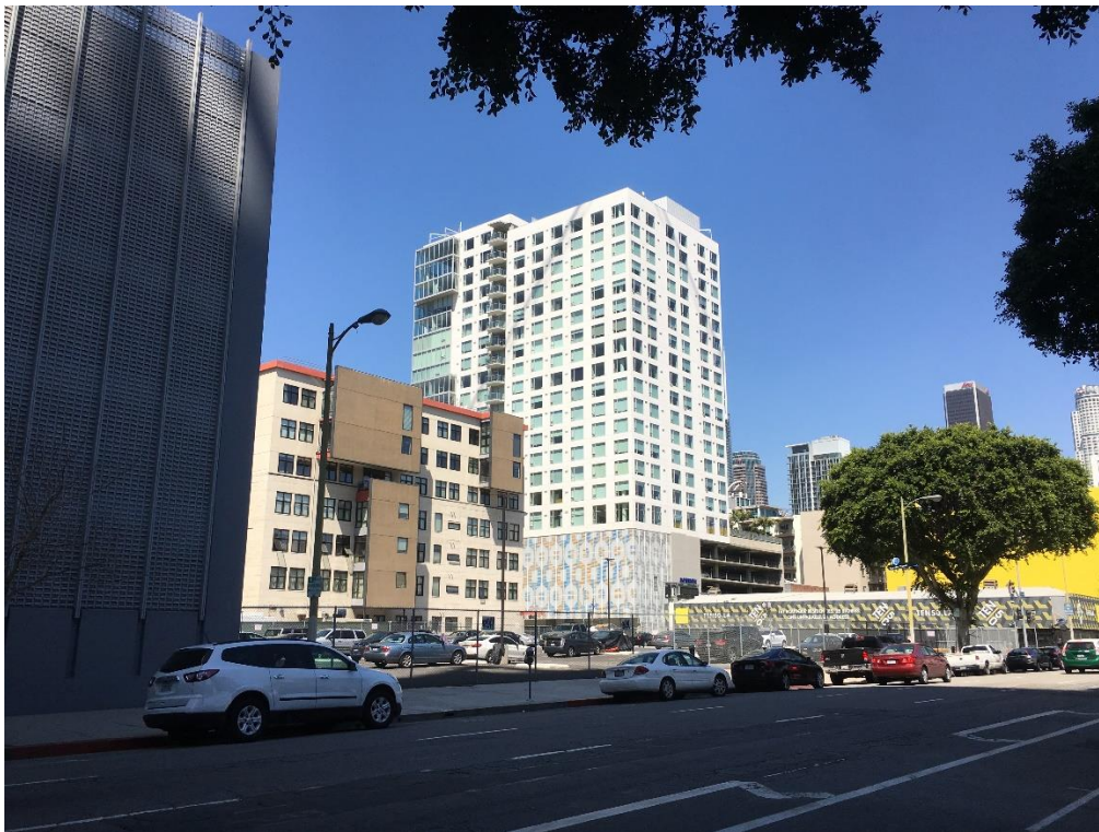
Photo 6: View of the project site from the South Corner (Facing north on Olive St.).
