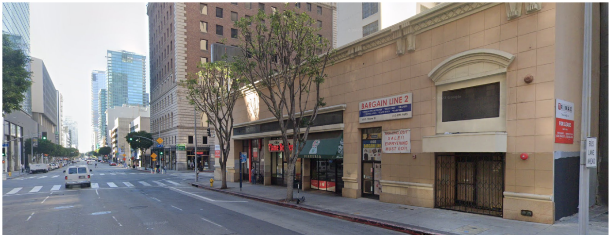
8. Southwest view of abutting uses on Flower st.
