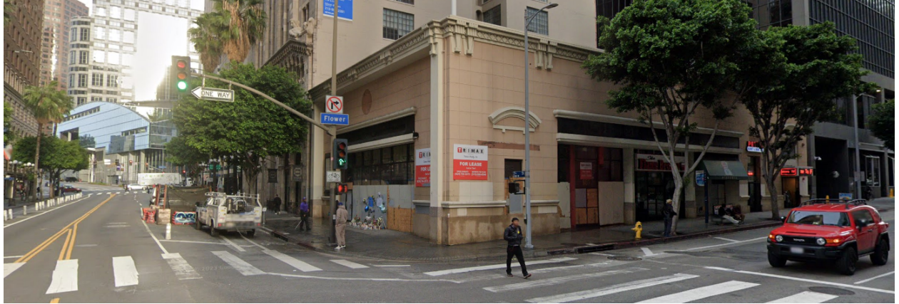
1. View of subject site
