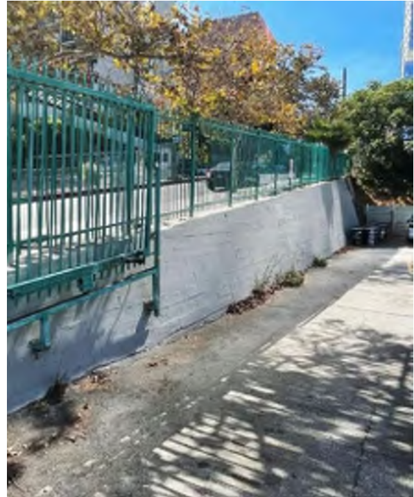
Figure 2: Existing Retaining Wall abutting 2nd Street ROW
