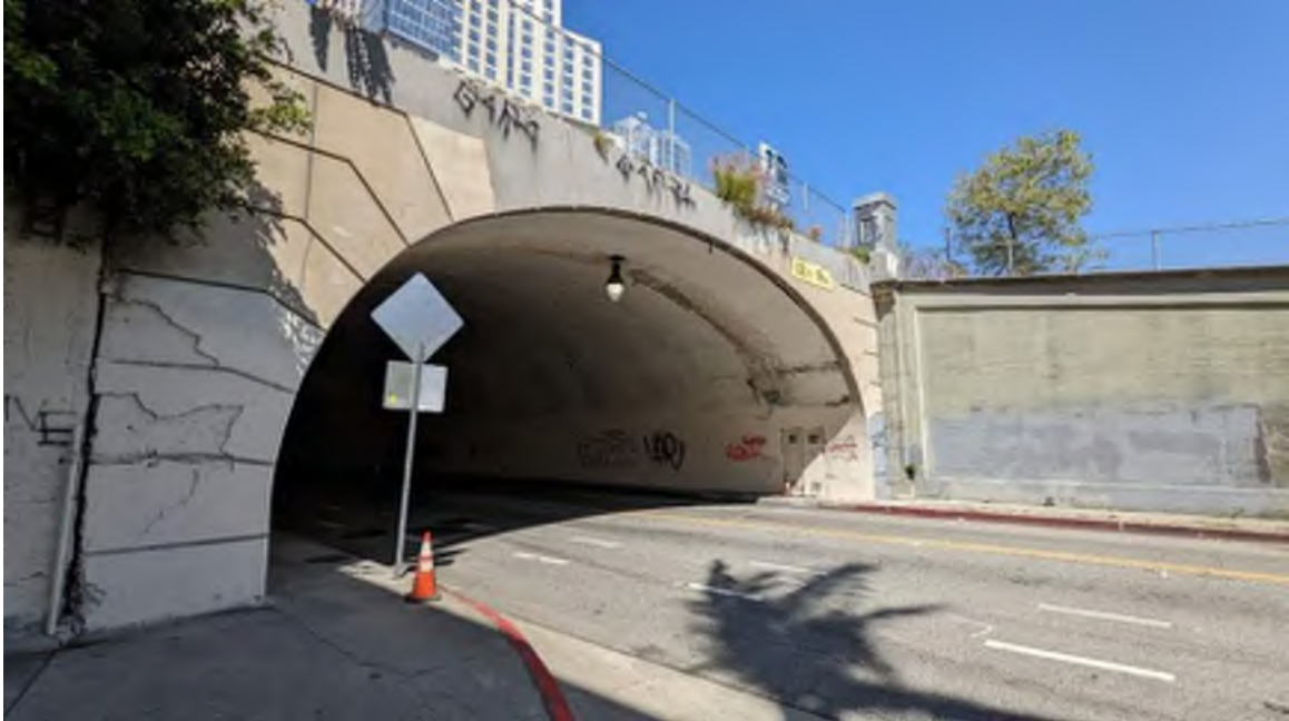
Photo 19: Facing northwest at 2 nd Street tunnel entrance from Hill Street
