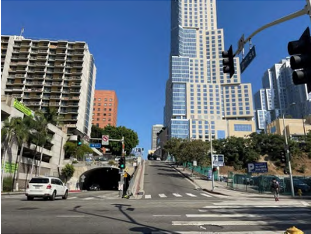
Photo 17: Facing northwest toward tunnel and 2 nd Street
