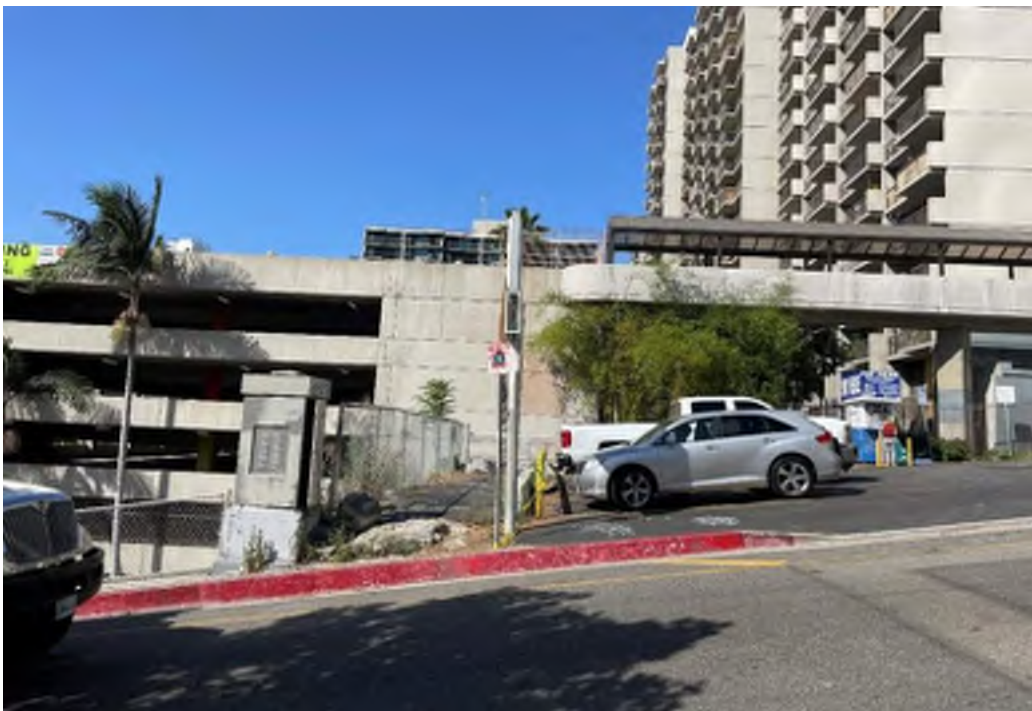
Photo 22: Facing northwest toward tunnel and parking lot adjacent to footbridge on 2 nd Street
