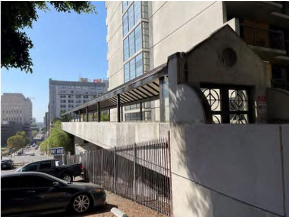
Photo 24: Facing southeast toward entrance of footbridge from Olive Street
