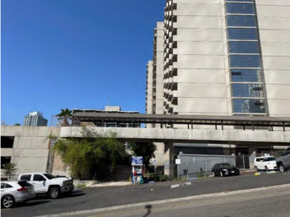
Photo 23: Facing northwest toward parking lot adjacent to footbridge on 2 nd Street
