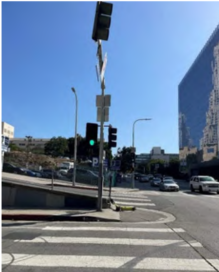
Photo 20: Facing northeast on crosswalk at tunnel and 2 nd street entrance
