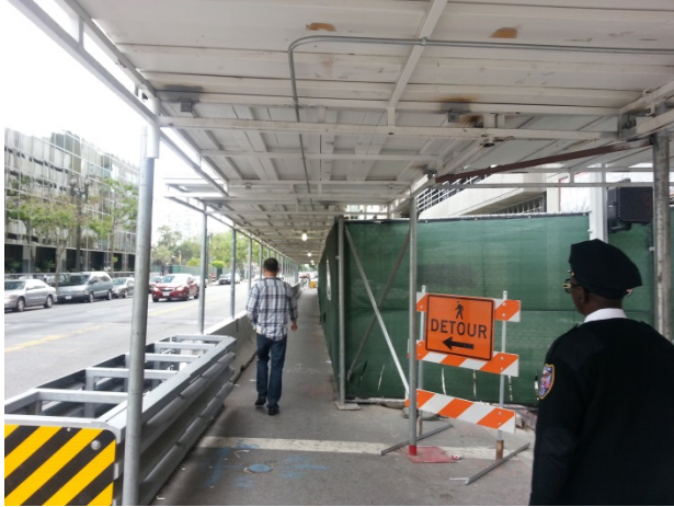
Picture above: Picture of pedestrian access along construction fence in front of new high-rise construction on Hope St. and 8 th St. This should be a requirement for all construction sites in Downtown LA.
