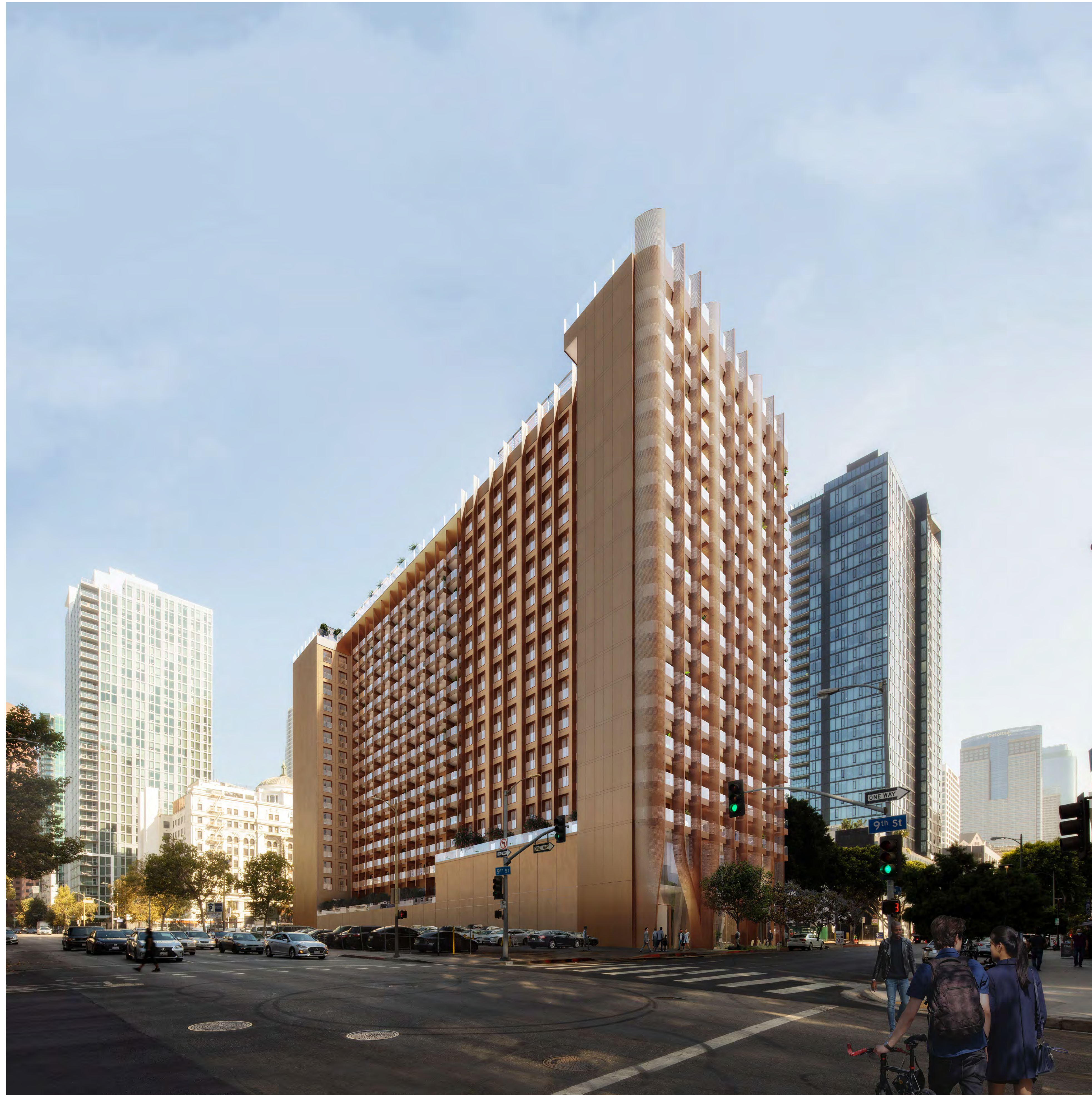
VIEW FROM OLIVE AND 9TH LOOKING NORTH
