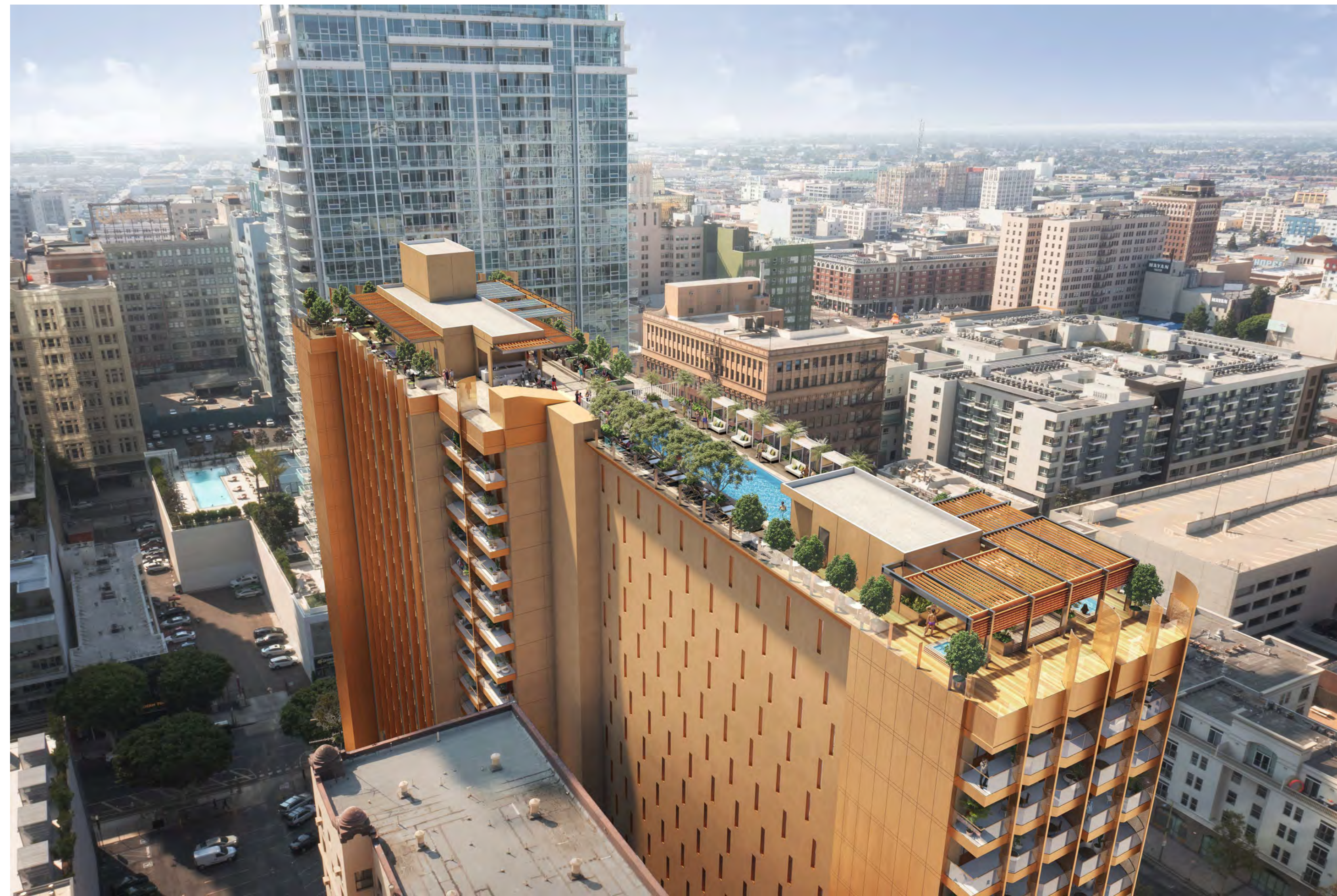
ROOF DECK AERIAL LOOKING SOUTH EAST
