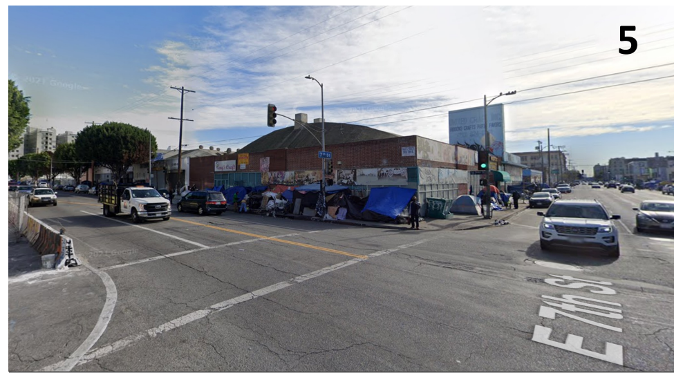
Figure 5 – View of the Subject Property from Southwest corner, facing northeast
